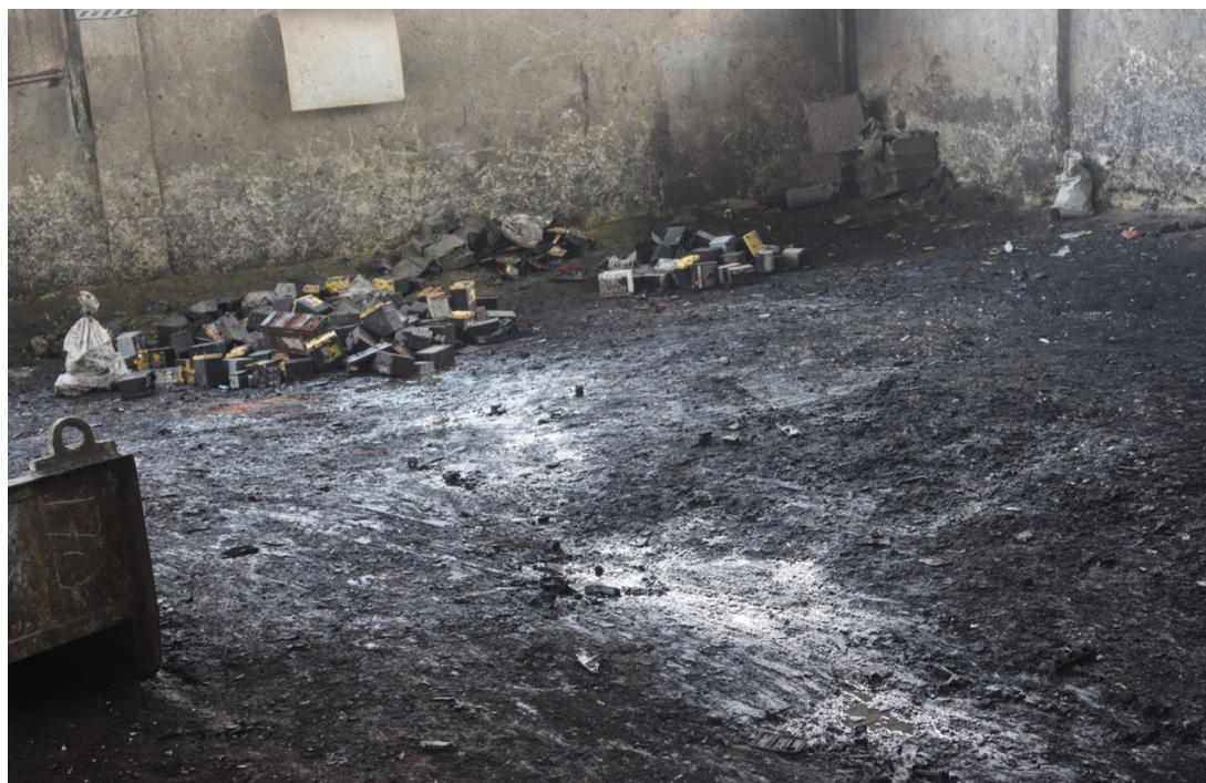
FIGURE 5. Battery breaking area with no functional system to capture electrolyte
