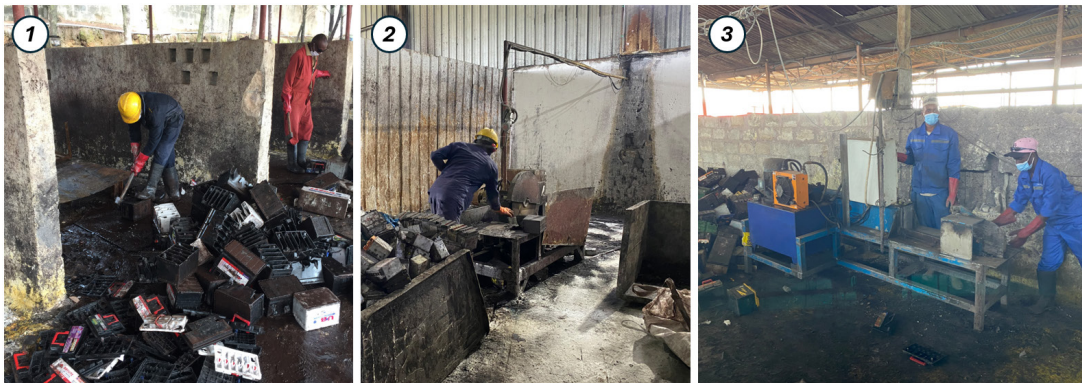
FIGURE 2. Battery breaking as commonly conducted in industrial ULAB recycling plants in sub-Saharan Africa
